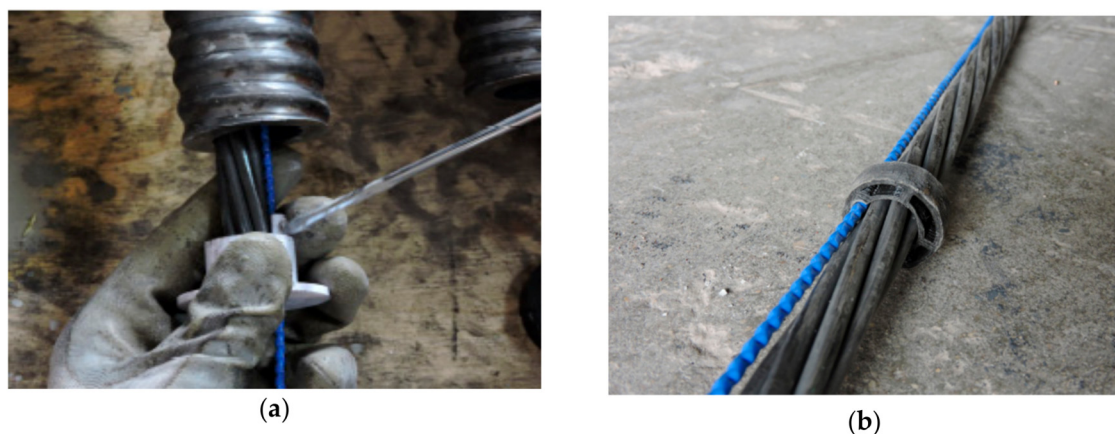
Figure 59. DOFS installation by means of plastic hooks for coupling the DOFS in an anchor's (a) extremity bar and (b) internal bar [139].
